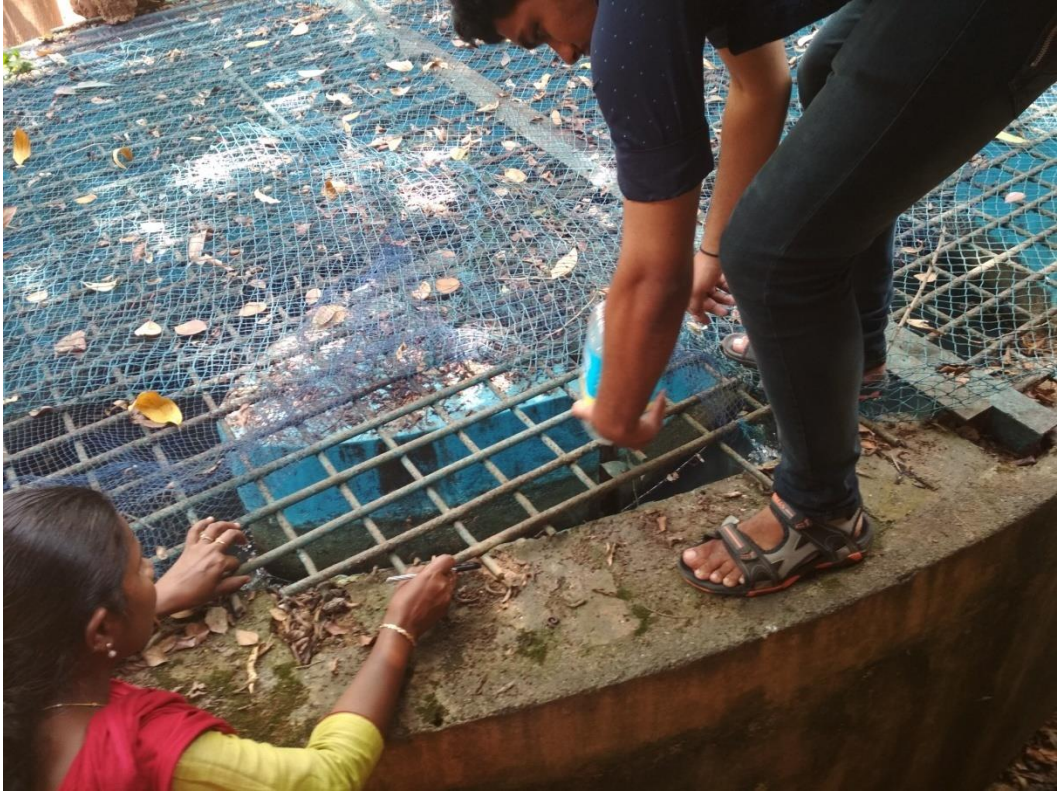
Chlorinating water tank
